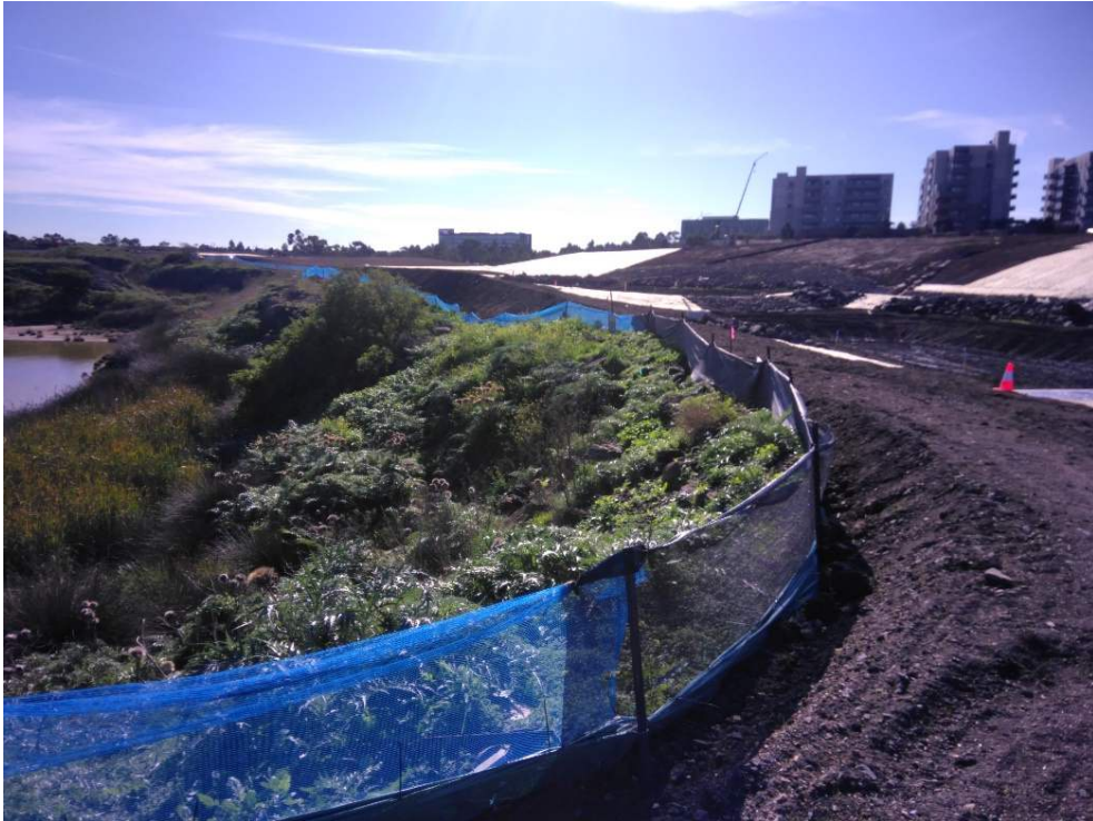
Photograph 3: Growling Grass Frog habitat proposed for removal has been retained.
