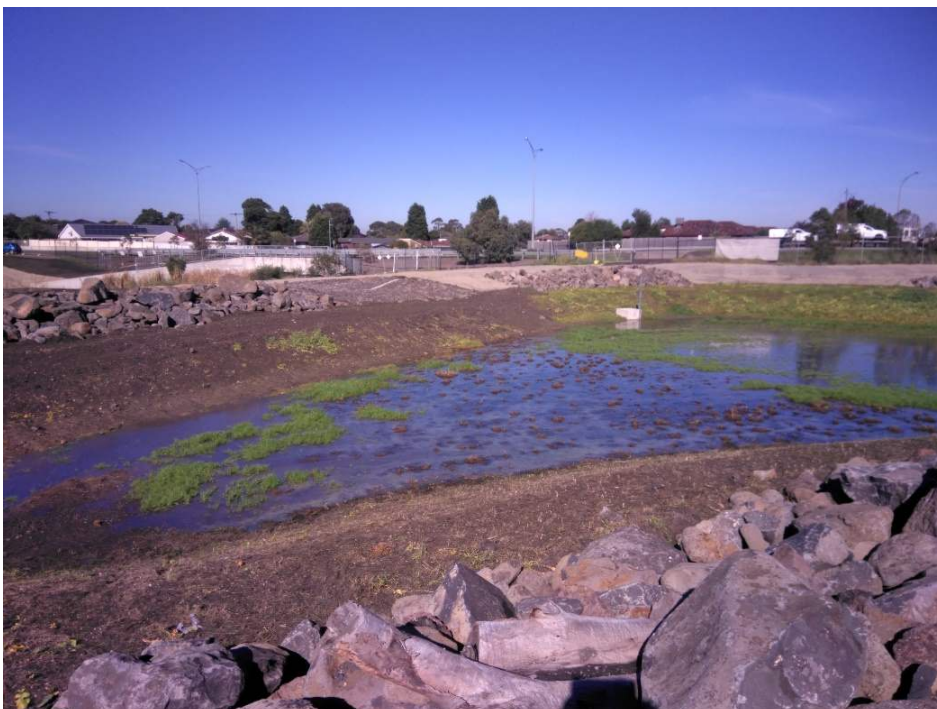
Photograph 2: Civil works completed in southern section of site.
